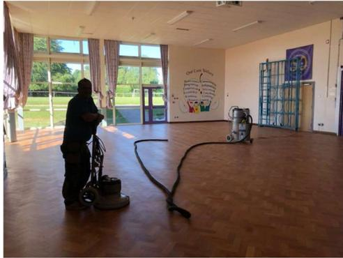
Work inside school has, in recent weeks, picked up pace and has been progressing well. We are delighted by how it is looking. The hall floor, which was damaged by the flooding, has been fully renovated and the beautiful original parquet flooring has been restored to its former glory.
